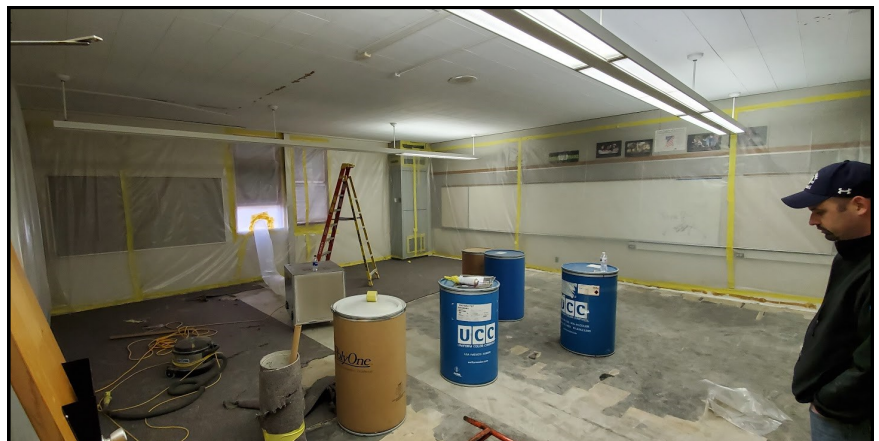
Initial work in late December included asbestos abatement work.
