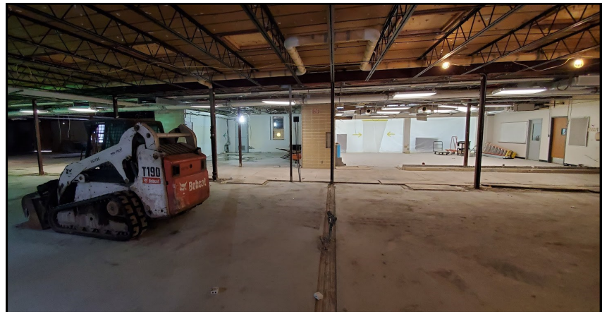
All interior classroom walls along with the hallway walls were removed.
